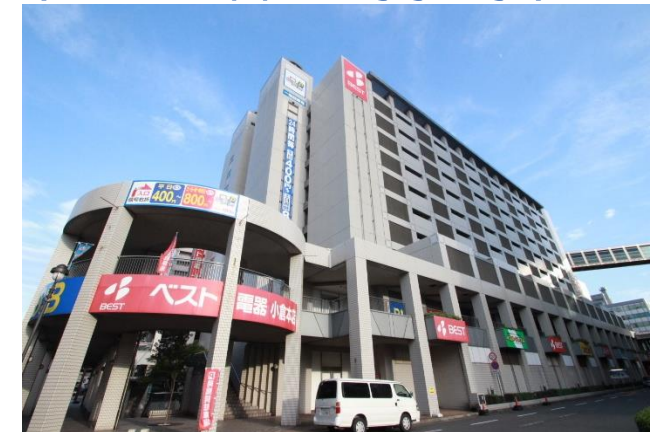
Multi-story, self-parking parking garage for 1,000 vehicles
