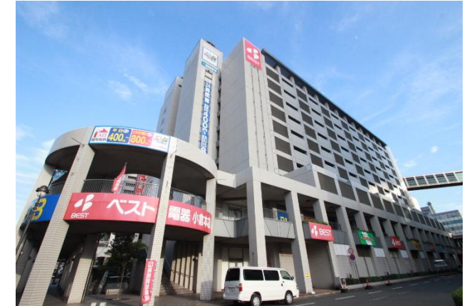
Multi-story, self-parking parking garage for 900 vehicles
